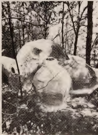
Igloo-like houses of urethane foam are formed by spraying over fabric and cable forms. Dwellings of almost any size or shape can be built in a matter of minutes.
